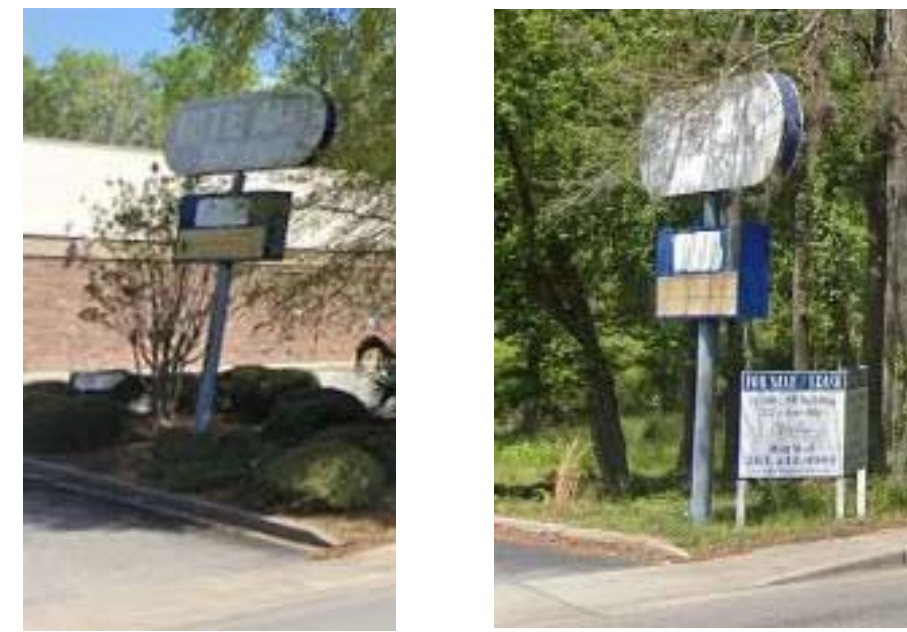
NOTE: DEMOLISH TWO (2) SIGNS ON SITE. LEAVE ELECTRICAL FOR POTENTIAL FUTURE SIGNS.
