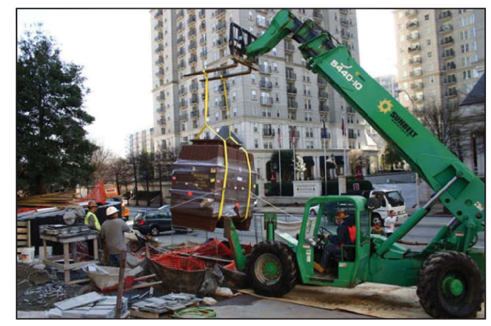
LIFTING FORK CRANE WITH DOUBLE STRAP SLING
