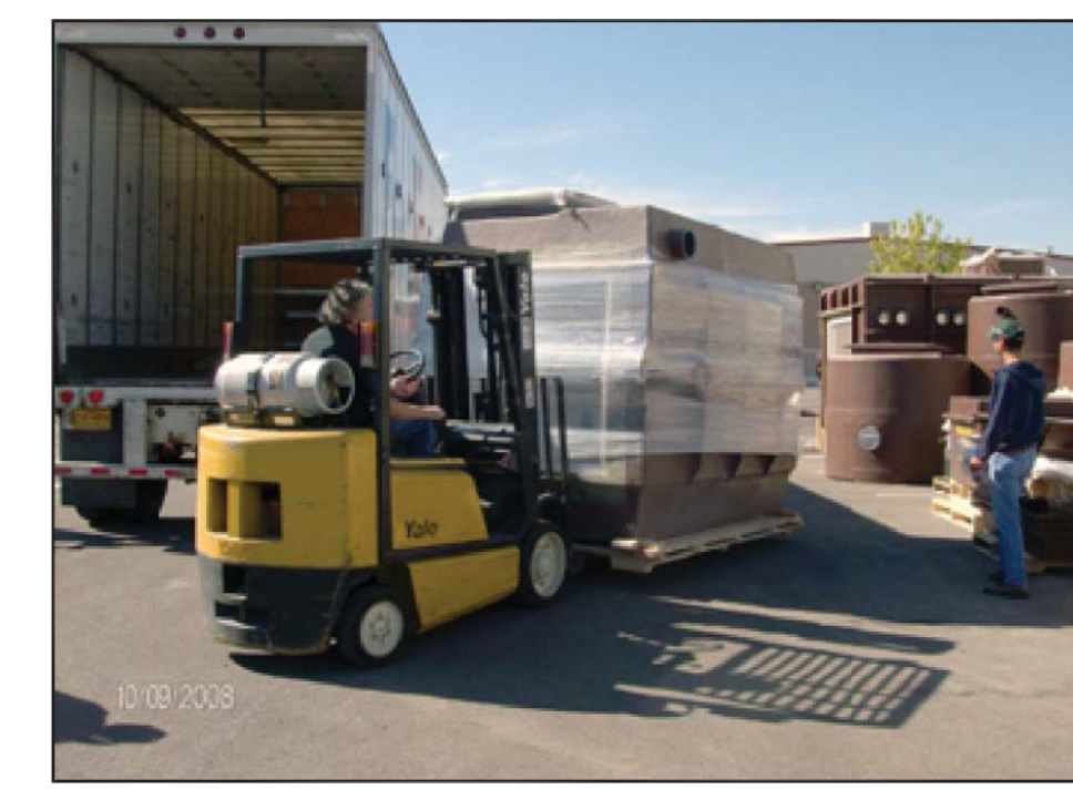
VAULT OFF-LOADED FROM TRUCK
