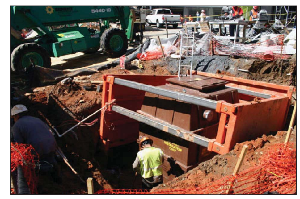
VAULT IN POSITION PROTECTED BY 'CAVE-IN' BARRIER
